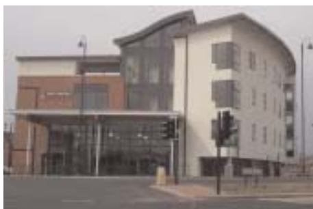
The New Charter building - Cavendish 249
